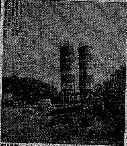
RMC plant setup
